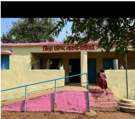
RENOVATION OF SCHOOL
