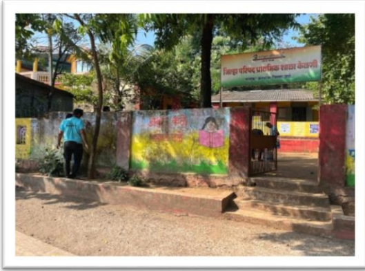
School Before Renovation
