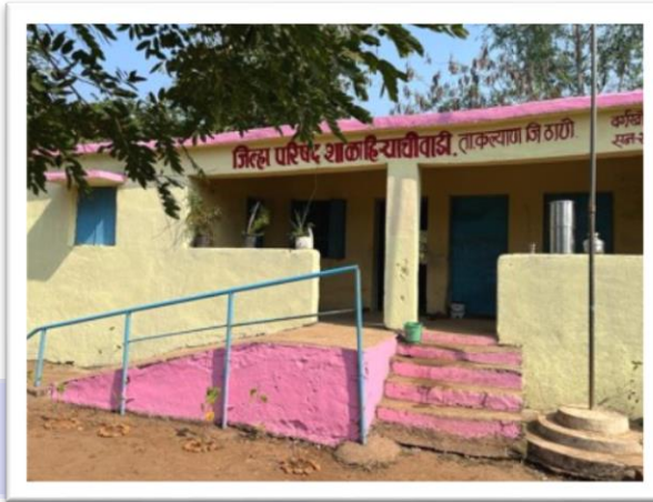
Picture after the renovation of the school
